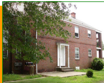
Fastow Apartment Building
